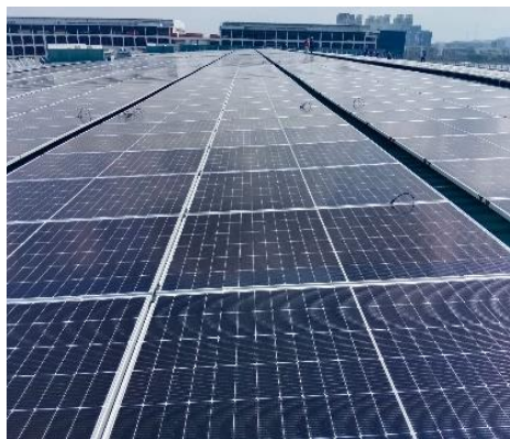
Solar panel installation at 34 Penjuru Lane
