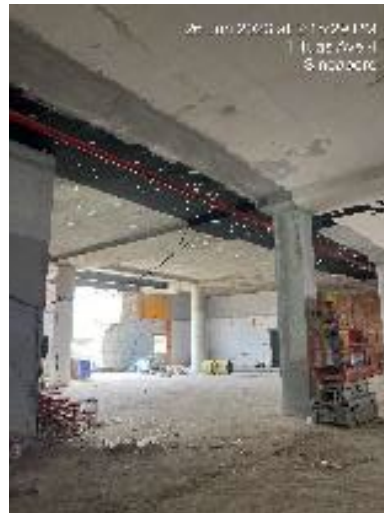
Touch Up Soffit of Slab @ L2
