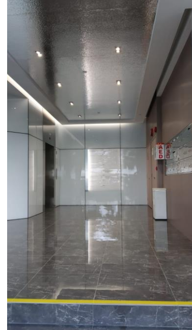
Upgrading of the lift lobby and drop-off area at 123 Genting Lane
