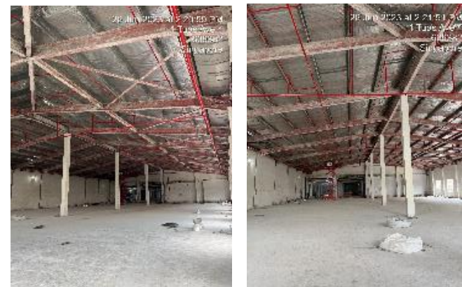
Vermiculite Removal and Cleaning
