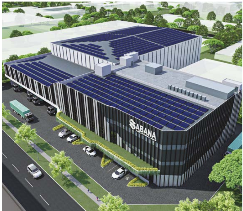
Artist's impression of the new 1 Tuas Avenue 4 which will target to obtain a minimum Green Mark Super Low Energy certification upon completion
