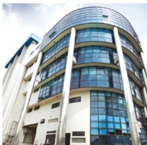
Modernisation of cargo lifts at 2 Toh Tuck Link was completed in 2022
