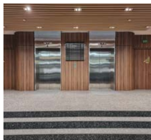
Upgraded passenger lift lobbies at New Tech Park
