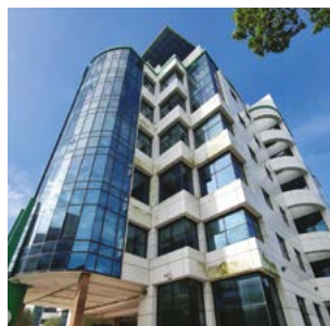
Installation of high-efficiency airconditioner chillers at 508 Chai Chee Lane
